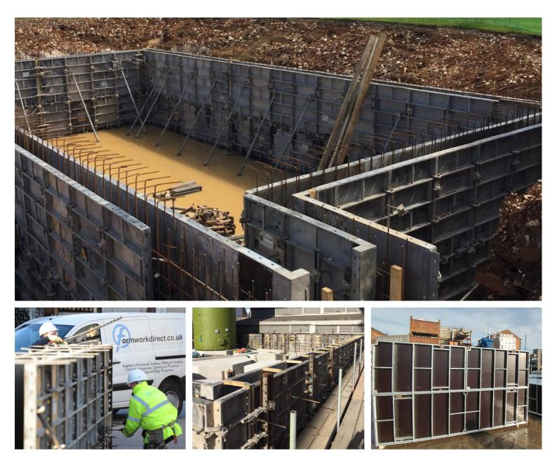
Frami Formwork is a man handleable formwork system that is perfect for foundations, bases and walls. The system has a robust galvanized frame and a safe working load of 50kN/M<sup>2</sup>.
