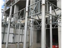
Aluminium components make High load capacity reduces the Compatible with H20 Timber amount of equipment required.
