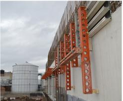
FDI Heavy Duty Soldiers are sturdy and extremely easy to build into beams of any length. FDI Heavy Duty Soldiers can be used in conjunction with Aluminium or Timber Beams and FDI Tie Bar in the construction of straight, curved and conical walls.
