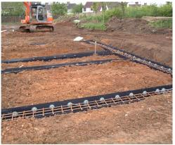
Beamform is disposable formwork for Ground Beams and Pile Caps. Polypropylene sheets provide contractors with a fast and effective means of forming ground beams and pile caps.
