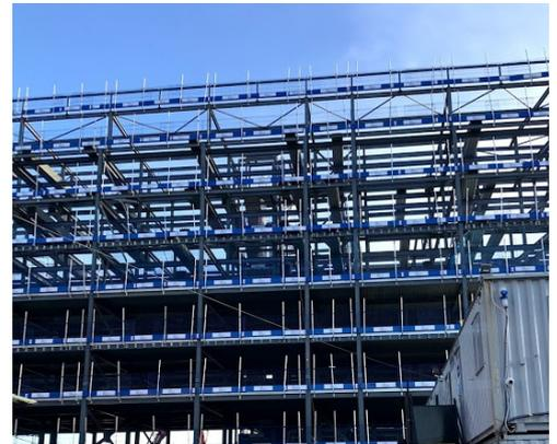
Combisafe edge protection systems have been specifically designed to meet the unique challenges of each construction technique, including steel frames, with a wide range of innovative attachments for the safe and secure fixing of barrier protection to beam edges, webs and faces. Combining a range of valuable benefits such as strength, durability, speed of installation and adjustability.
