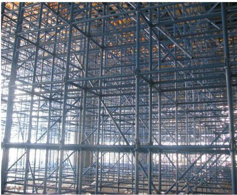
Up to 74 kN leg load results in larger grids with less materials being used.
