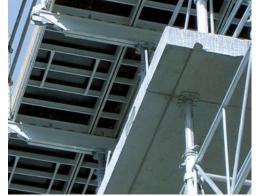
Assembling panels and beams from below the soffit lowers the risks associated with working at height.
