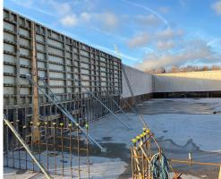
Alkus panels are solid plastic formwork panels made from aluminium reinforced polypropylene that are typically used for wall formwork and special structural elements because of its excellent flexural strength.
