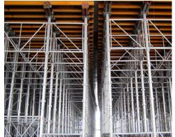
With a leg loading capacity of up to 120kN per leg, fewer supports are needed, streamlining the setup.
