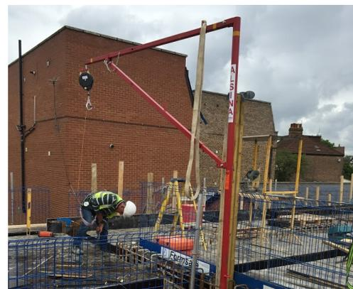
Alsipercha is a fall protection system that provides effective overhead protection for those who are exposed to falls when working at heights.
