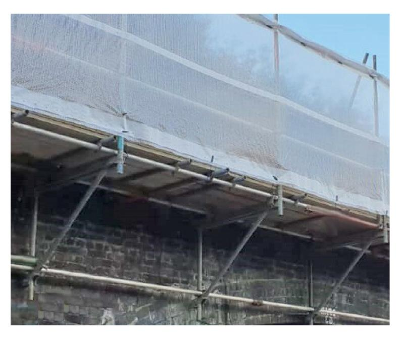
CL25 Access Brackets provide safe access and formwork support for lifted pours.
