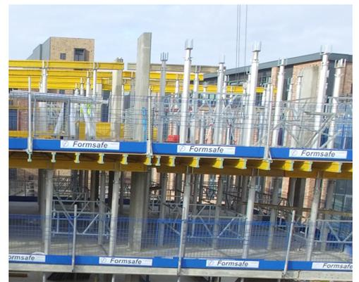
Combines guardrails, toeboard and debris mesh in one product
