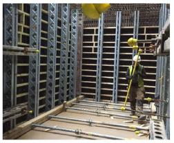
Lighter than timber which enables faster and larger formwork assembly
