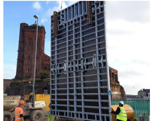
The FD Max panel is a heavy duty wall formwork system capable of taking loads up to  $90\text{kN m}^2$ . The system is used in all areas of construction i.e., civil engineering, building and infrastructure projects of all types.
