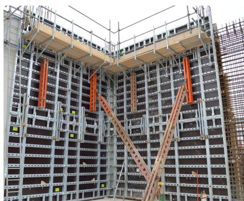
Capable of taking loads of up to 90kN
