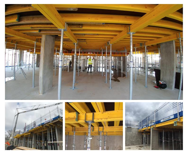
Formflex is a temporary works system to facilitate the forming and support to suspended concrete slabs
