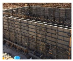
Capable of taking loads of up to 50kN
