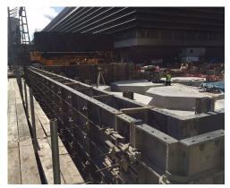
Manhandleable steel framed formwork for foundations, walls and columns.
