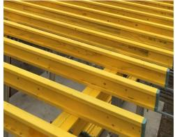
Formwork Direct H20 beams are made of Spruce wood.
