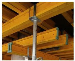
The web is made of 3-ply solid wood panel, ensuring high carrying capacity and durability in all climate zones
