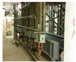
1000 kN permissible load makes Megashor ideal for heavy duty falsework, and façade retention
