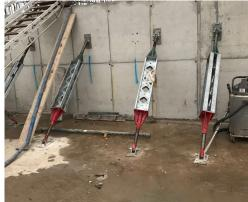
Megashor Props are ultra high duty modular props designed to handle high loads.
