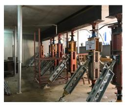
Can be assembled into props, towers and trusses of almost any length due to the variety of sizes and accessories
