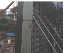
Features telescopic design and Versatility enables options for faster length adjustment due to rough setting and fine tuning.
