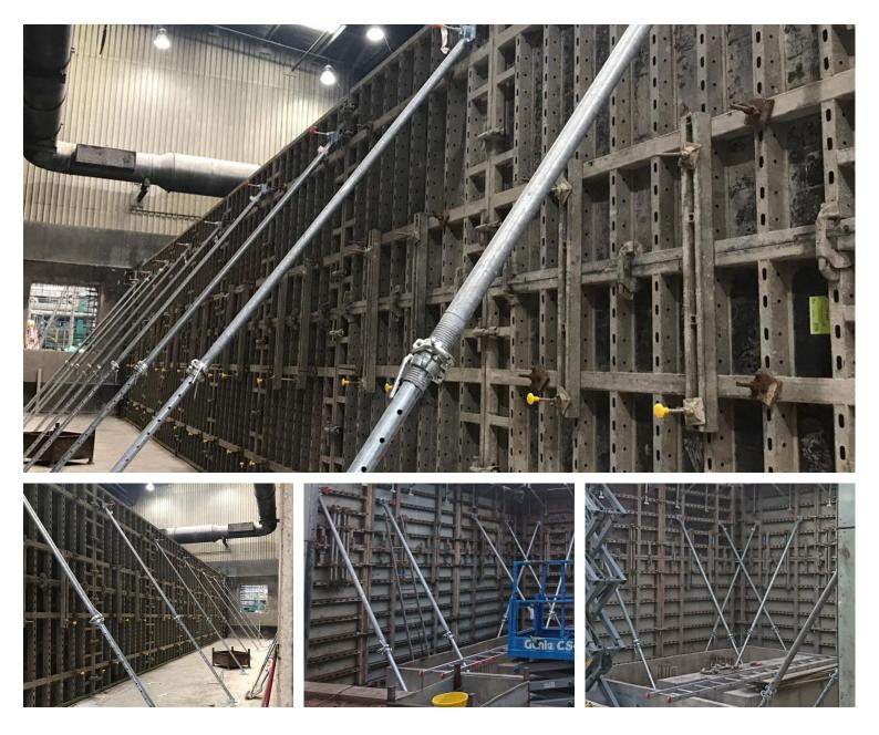
Formwork Direct push pull props can be used in all possible cases to support prefab elements, standard system formwork and steel during construction.
