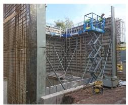
Ideal bracing solution for formwork panels.
