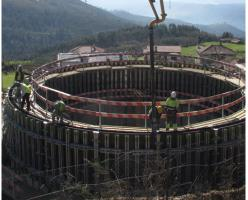
The FD Max Roflex Circular Formwork System is the perfect solution for projects that require curved wall sections such as silos, waste water treatment plants, access ramps to multi story car parks and other circular structures.
