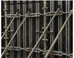
Precise radius adjustment using turnbuckles.
