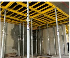
Fastdeck is a modular slab formwork system with only two basic components, props and panels. This enables fast and safe erection with minimal labour.
