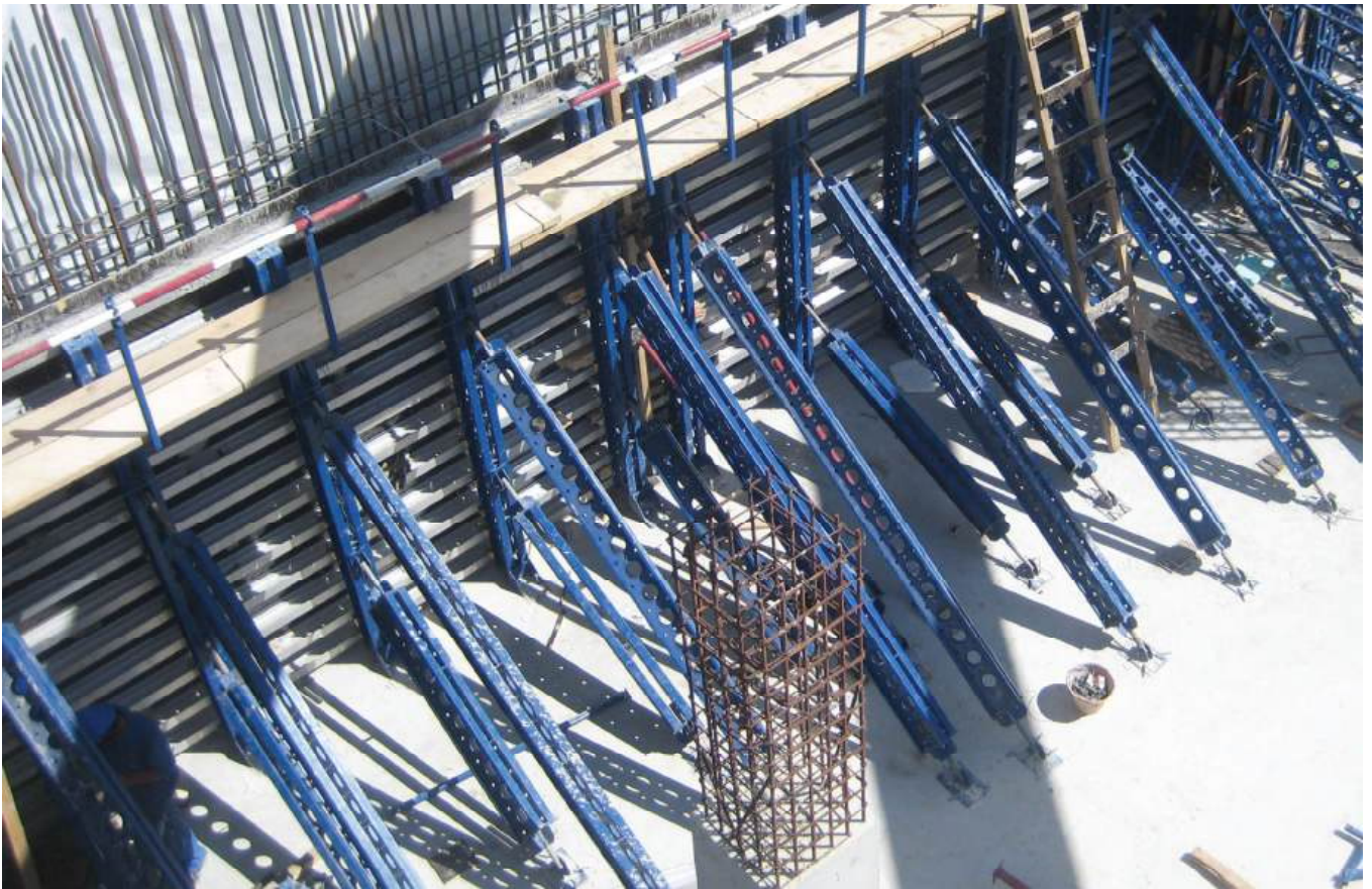
Vertical Struts - Buckling About the Y-Axis
