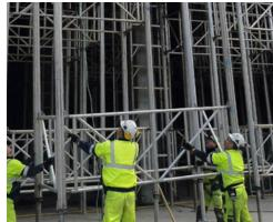
Unique locking ledger frames located at any position on the outer leg
