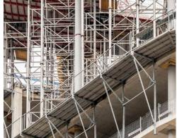
GASS is a high-capacity, lightweight shoring system designed for simplicity and speed and suitable for a wide range of projects from straightforward square slabs to complex angled slabs.
