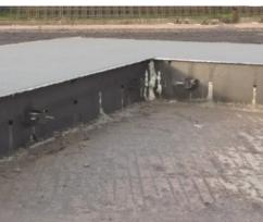
Formwork Direct Roadforms consist of a channel-shaped steel section, normally 3 metres in length and either 100, 150 or 200 mm in depth, with 3 fastening brackets fixed to the back edge and a sliding tongue-fitting that enables adjacent section to be linked together.
