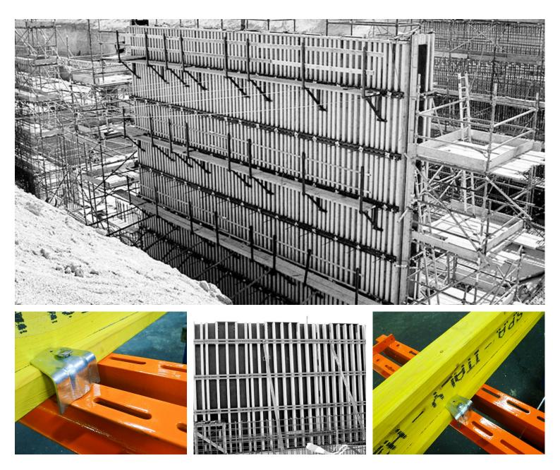
WS10 Multiform is a Large Area Formwork System that is prefabricated dependent on project specifications enabling it to handle many different types of task as the shape, size, tie-hole pattern and form-facing of the elements can be adapted to suit any requirements which in turn permits any pouring rate as it can be easily dimensioned for any fresh concrete pressure.
